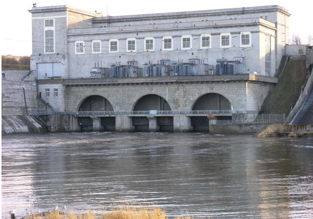
Figure 9. The hydropower station on Narva River has three turbines
